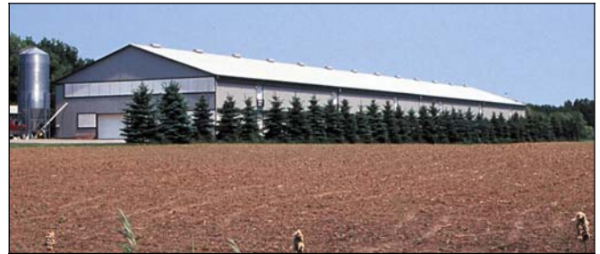
FIGURE 5. A tree windbreak around livestock production facilities helps filter odours and improves the effectiveness of separation distances by creating a visual barrier to the adjacent barn.
