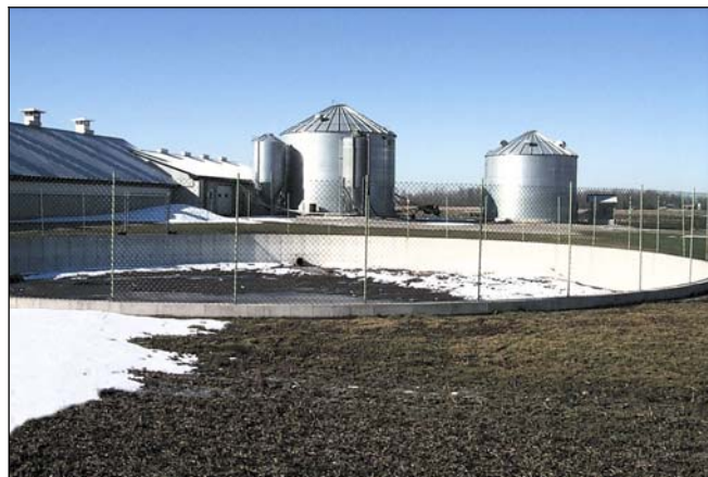
FIGURE 2. Storage structures are used to contain liquid manure until field conditions permit application and at a time when the crop grown can best utilize the nutrients.
