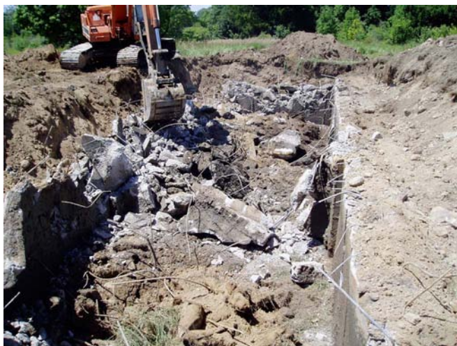
Figure 1. This unused manure tank is no longer environmentally sound. The excavator is in the process of demolishing and burying the structural materials on-site.
