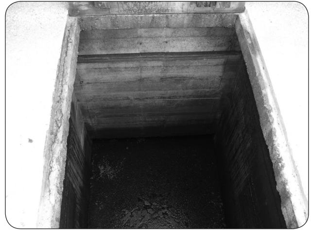
Figure 3. Pump-outs with baffles will cause the head spaces in unvented storages to become pressurized once the manure level rises above the bottom of the baffle.
