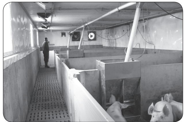
Figure 1. All rooms over manure storages should have ventilation operating at all times.
