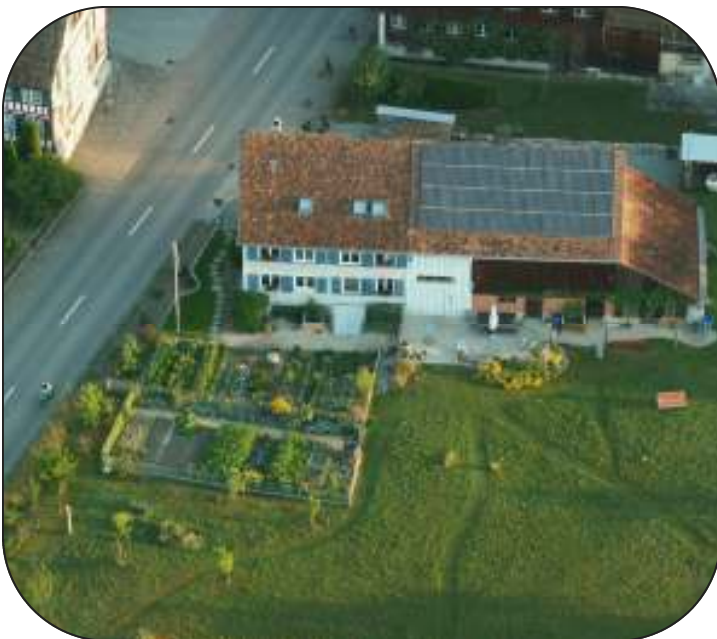
Figure 1. Solar photovoltaic installation on residence Hohentannen
